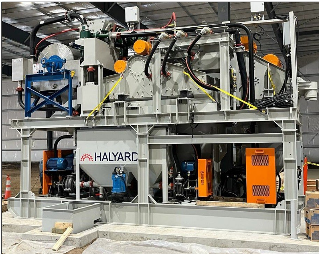
Commissioning begins for a dense media separation plant at Vital's Saskatoon rare earths extraction facility
